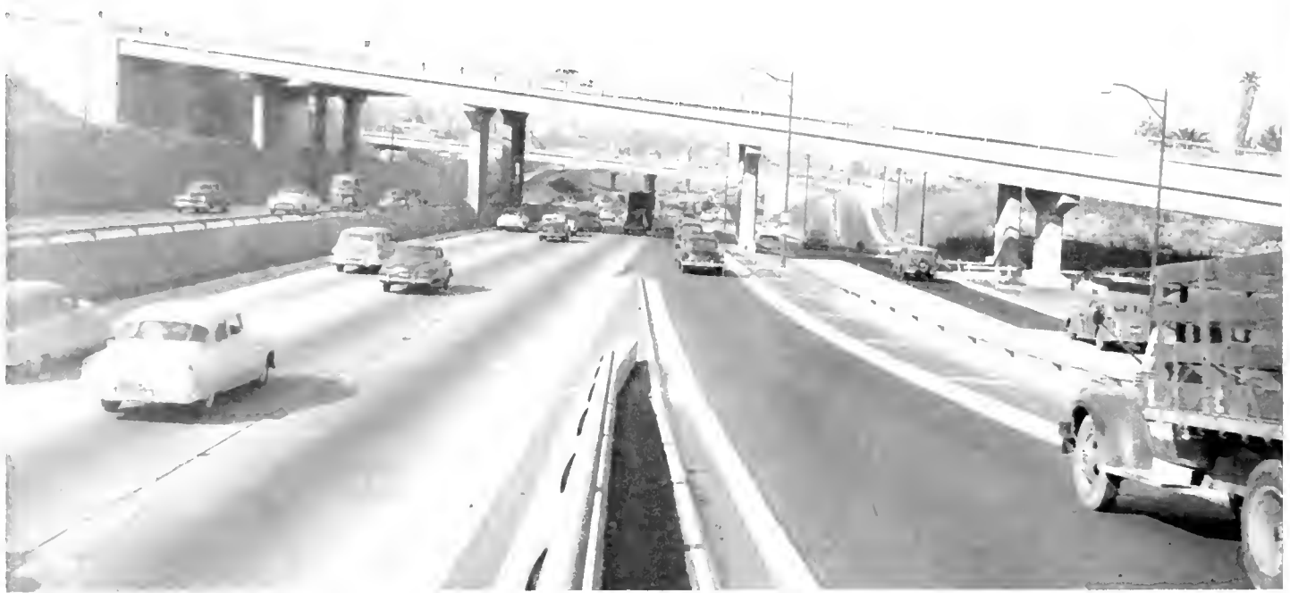
Looking northerly along completed Harbor Freeway, showing normal traffic use. The two bridges in foreground are for Fourth Street traffic. When cooperatively financed $1,400,000 construction contract now in progress has been completed for extending Fourth St. from Flower St. to Hill St., Fourth St. and Third St. will be put into operation as a pair of one-way streets similar to the one-way operation of Fifth and Sixth Sts., and Eighth and Ninth Sts.
